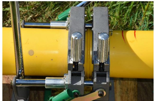
PA 12 butt fusion in the field in Henderson, KY. The bead formed during fusion is stronger than the pipe itself once it cools.
