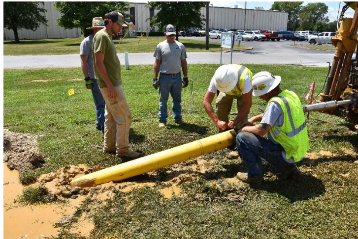
Teel's PA 12 pipe being pulled through HDD hole
