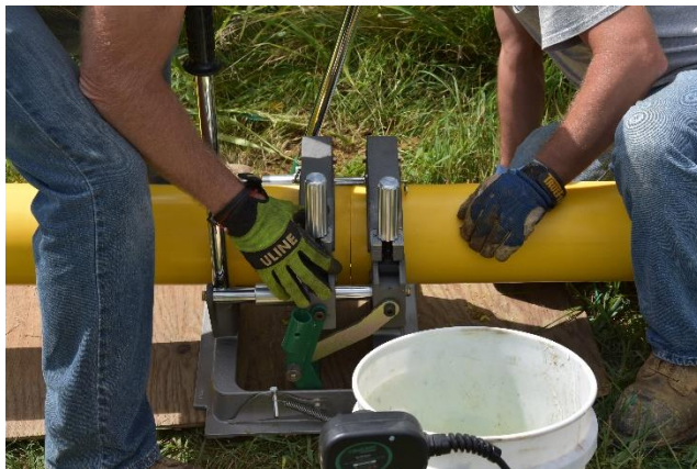
PA 12 butt fusion in the field in Henderson, KY. The bead formed during fusion is stronger than the pipe itself once it cools.
