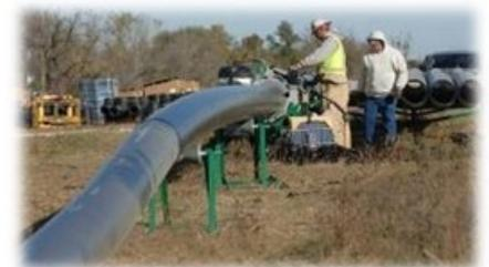
machine clamps to match the pipe OD to be butt fused.
