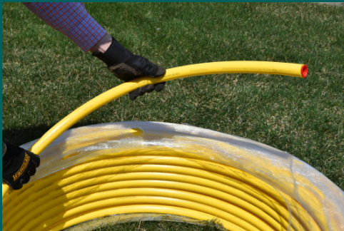
Locate inner pipe and pull out.
