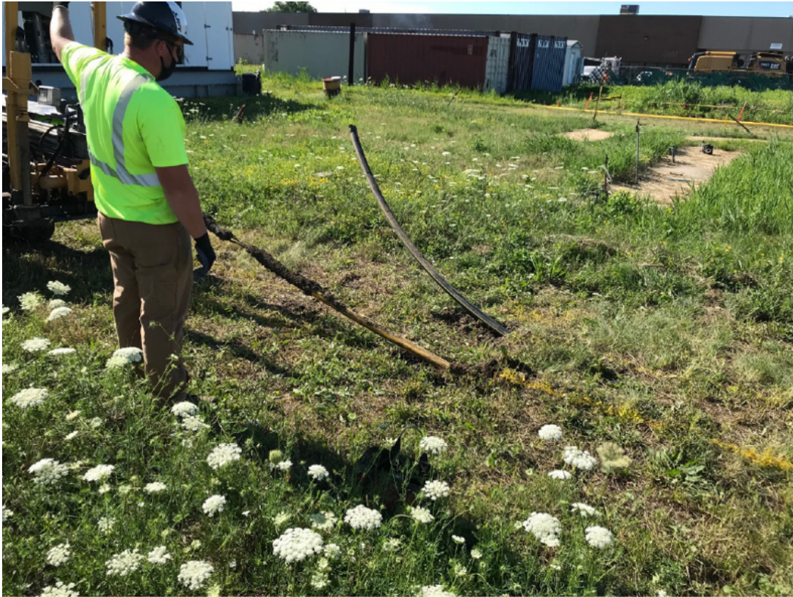
Figure 12: Field test HDD installation in progress
