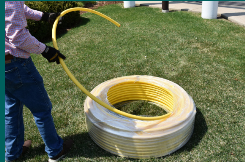
Continue pulling in direction the pipe is pointing.
