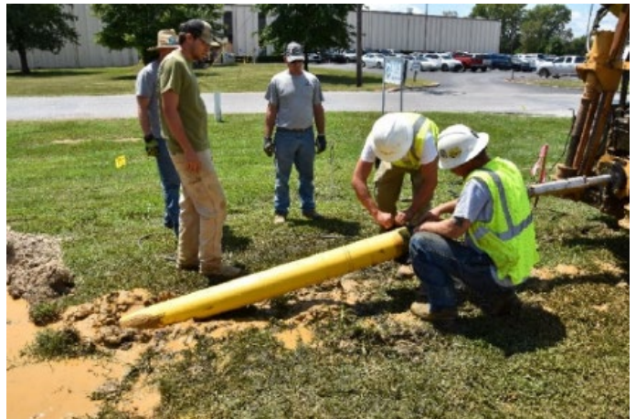
PA 12 installation in Henderson, Kentucky
