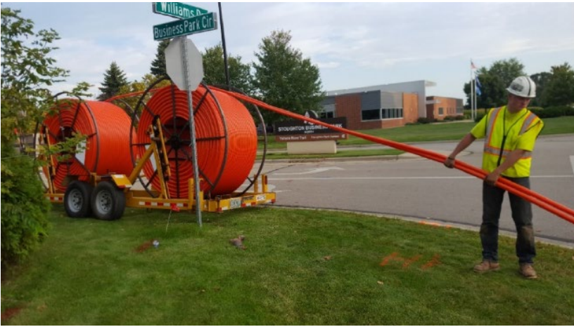
Installation of Teel Conduit by Alliant Energy in Baraboo, Wisconsin
